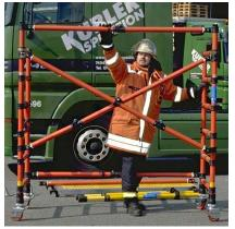
4. Push up the cross and diagonal brace simultaneous until the latches snap
